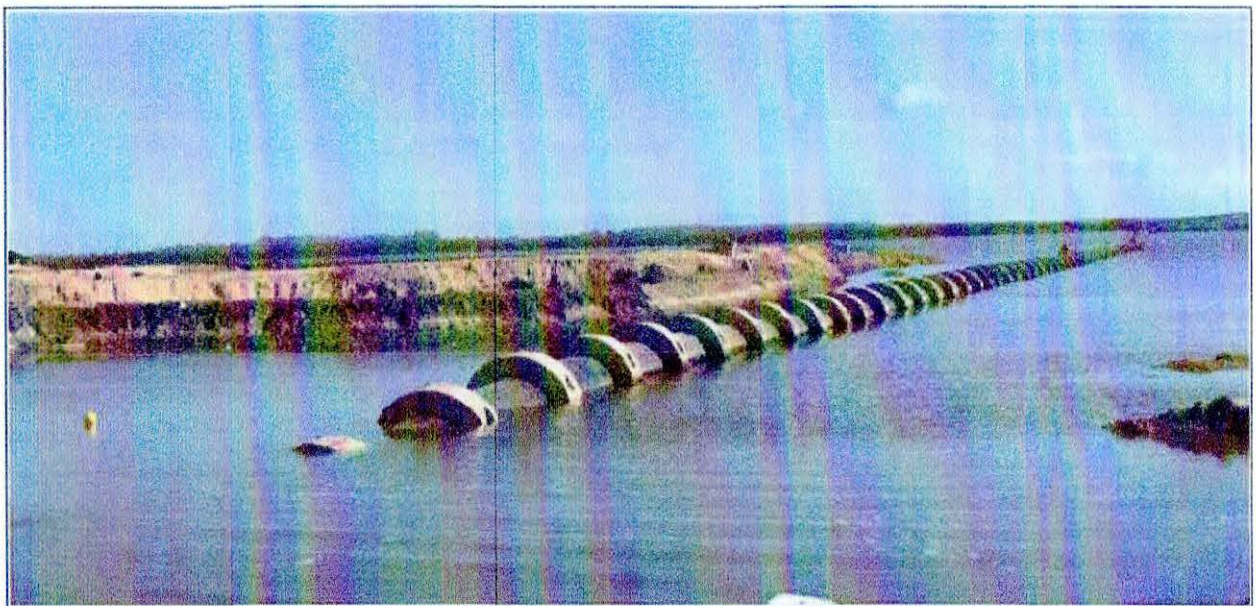
Figure 21: Step 4 - Submersion by water filling/air evacuation - copyright PipeLife Norge AS
