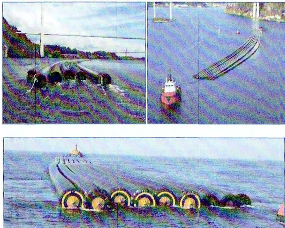
Figure 16: Transport of Long Lengths of Pipe to Site – copyright PipeLife Norge AS
