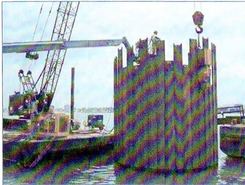
Figure 11: Construction of Cofferdam
