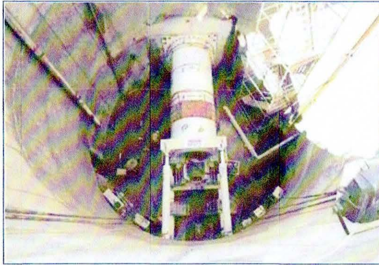
Figure 8: Micro-Tunnelling Machine Launch Shaft
