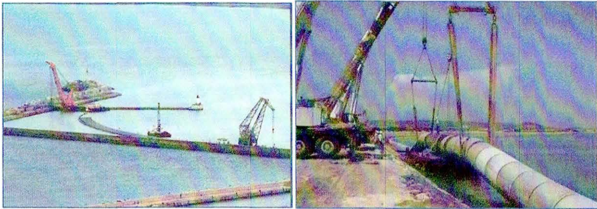
Figure 18: Typical Ballasting and Pipe Assembly Location off Quay wall
